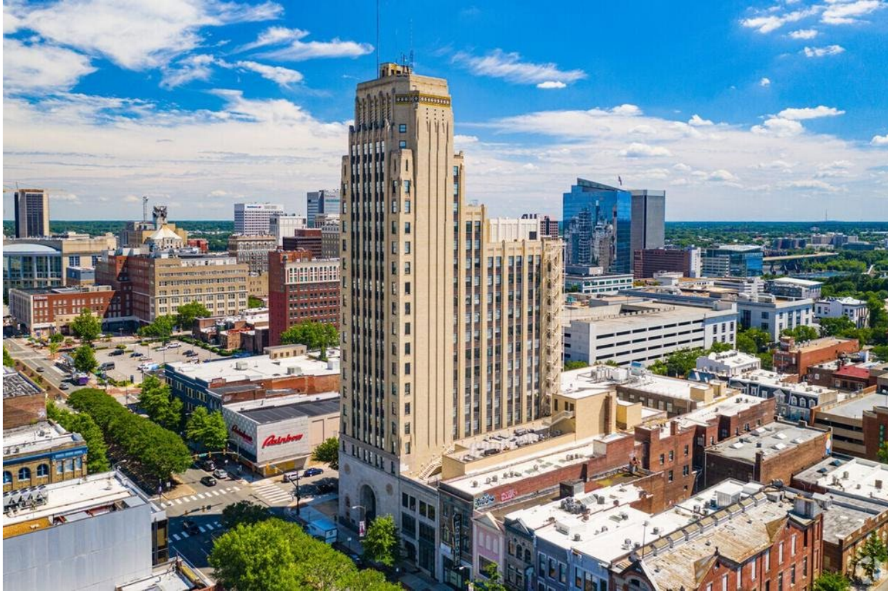
Deco at CNB Richmond, Virginia
